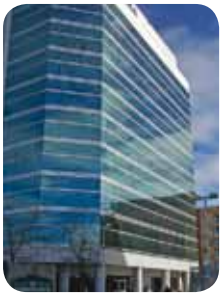
CANADA Adobe Tower
